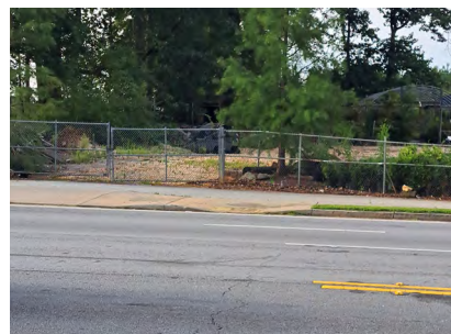
Curb Ramp at Intersection with Scarbrough Dr Shows Previous Midblock Crossing
