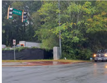
Arabia Mountain PATH Trail at Crossing with Covington Hwy Does Not Have Pedestrian Crossing Signal
