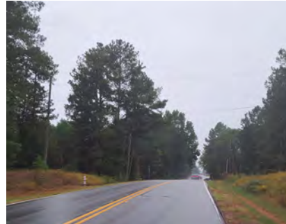
Between Rockland Rd and Mall Pkwy, the Corridor Has One Travel Lane in Each Direction with Drainage Ditches on Either Side
