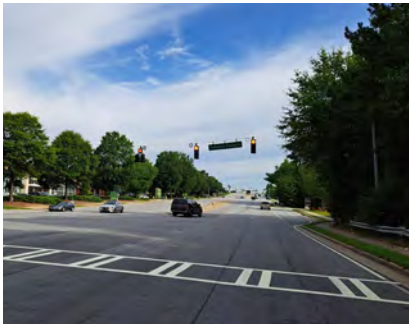
Turner Hill Rd from Mall Pkwy to I-20 Has Three Lanes Each Direction but also Sidewalk Connectivity
