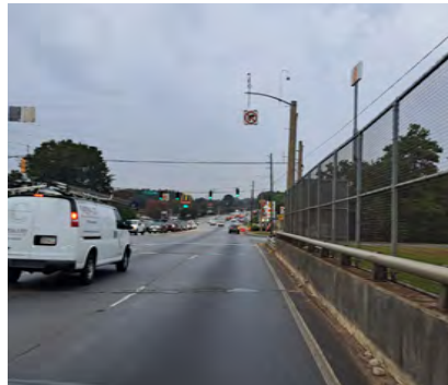
View North from Bridge over I-20; Sidewalk Only Present on West Side of Bridge and not East Side
