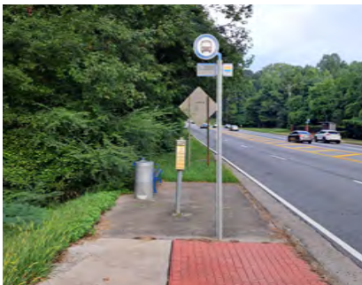
Dead-End Sidewalks Are Common Along Covington Hwy, Including West of a Bus Stop Across from Strathmoor Manor Dr
