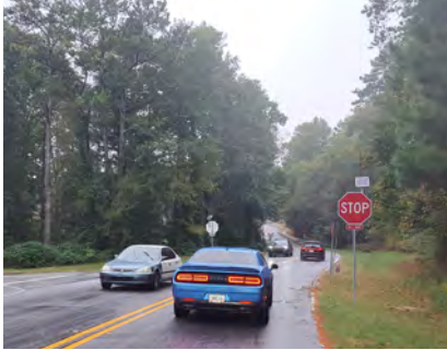
Turner Hill Rd at Rockland Rd is an All-Way Stop with Illuminated Stop Signs
