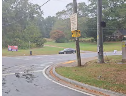
ADA Compliant Gaps Present on Southeast Corner of Intersection with Covington Hwy but No Sidewalks
