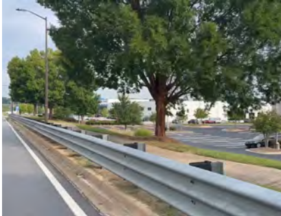
Guardrail Separates Sidewalk from Travel Lanes on north side of Mall Pkwy from Stonecrest Trce to Wesley Stonecrest Cir
